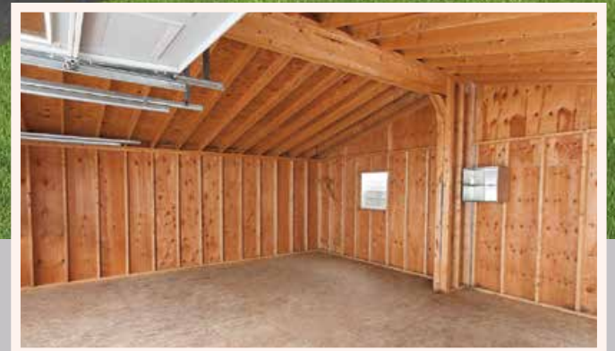
Interior of Double Wide Garage
