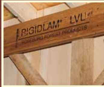
Glue LAM LVL header for increased snow loads and hurricane regions
