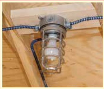
Vapor proof lights with die cast guard
